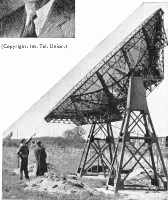
Radio-astronomy: two spaced paraboloids for producing a multi-lobed interference pattern (Cambridge University).
